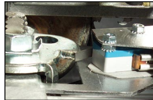
Check drain safety switches.
